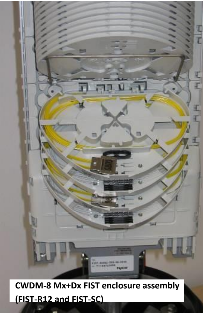
CWDM-8 Mx+Dx FIST trays (2 pcs FIST-R12)
